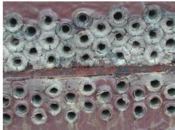
Fig. 1: Clogged H<sub>2</sub>S cooler: mud and scale.
