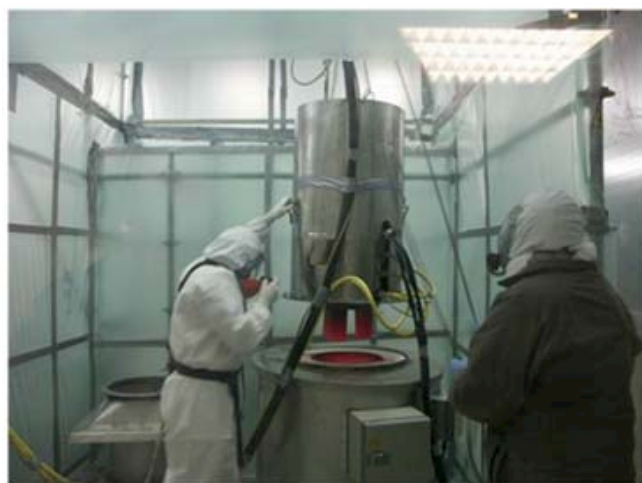
Figure 5: Operation of prototype unit at experimental waste centre (CMS, France).
